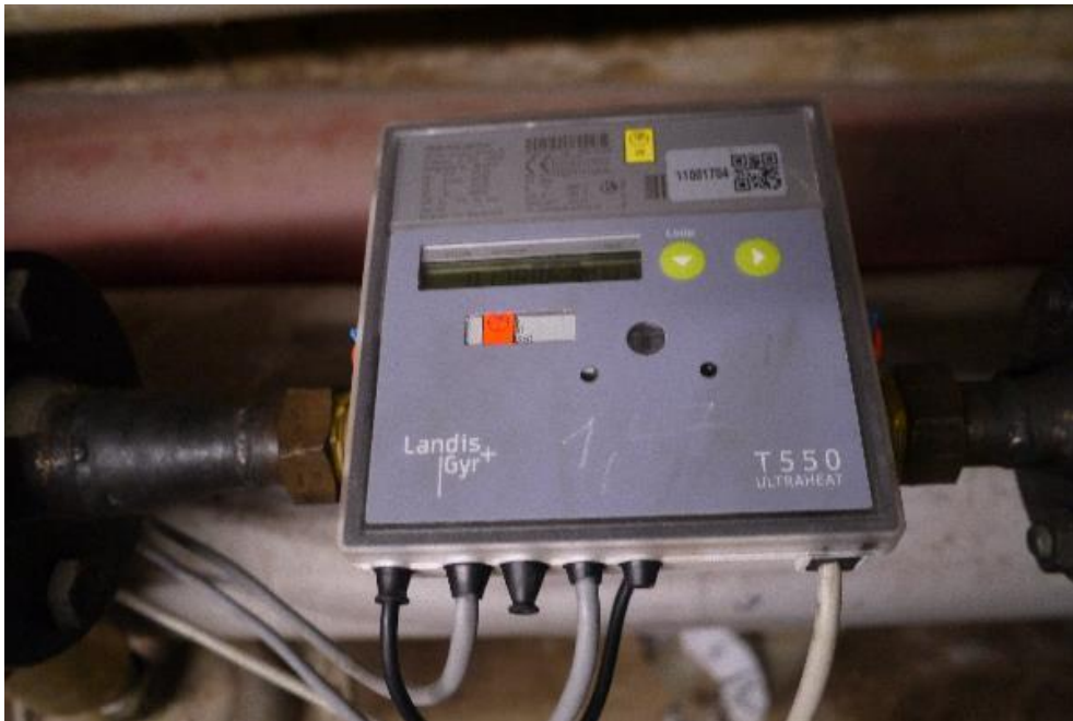
Figure 126: Heat meter
