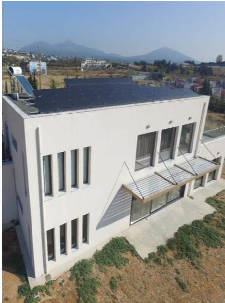
Figure 21: Smart House South view
