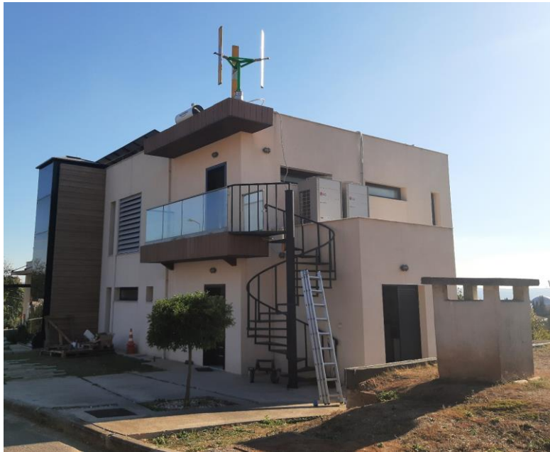
Figure 23: VAWT installed at CERTH's Smart House
