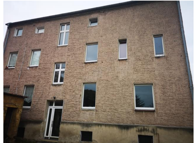
Figure 41: View on south side windows
