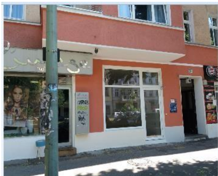
Figure 125: Renewed PVC windows
