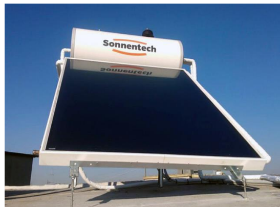
Figure 22: Solar thermal collector with hot water storage tank
