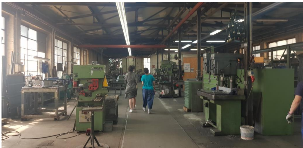
Figure 60: Case Study #3 - View of the roof of production hall 1
