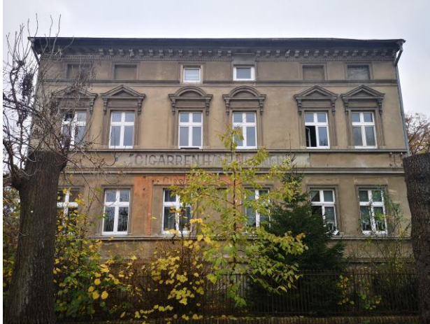
Figure 42: View on south side windows
