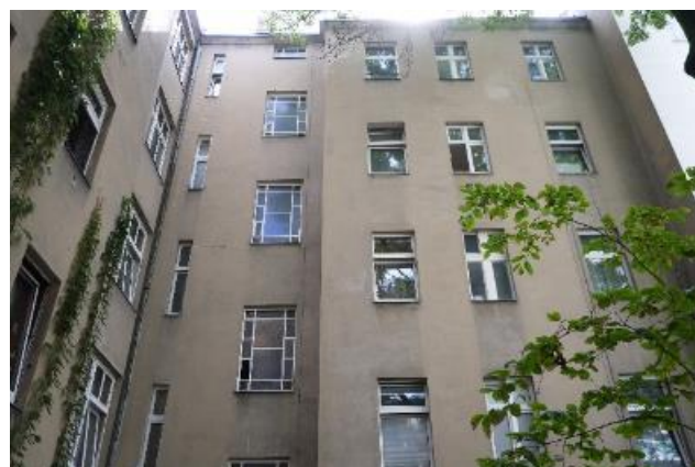
Figure 116: View from the street side and from the backyard Case Study 6
