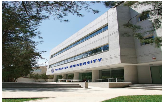
Figure 71: Frederick University New Wing façade
