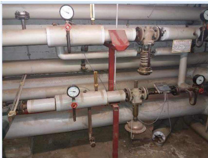
Figure 124: District heating transfer station
