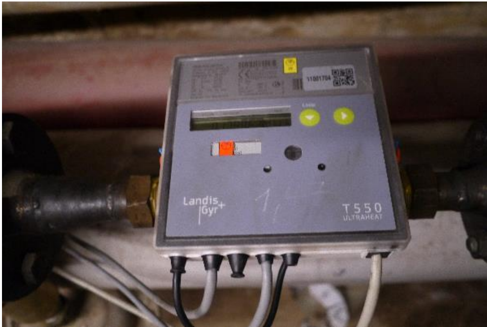
Figure 122: Heat meter
