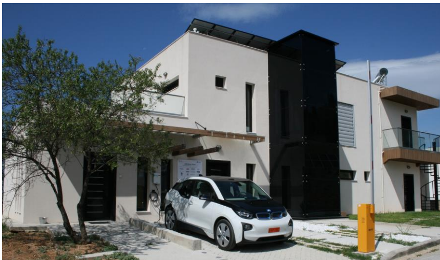
Figure 35 nZEB Smart House DIH
